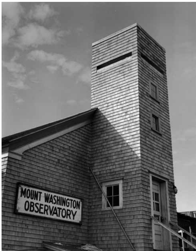
In 1937, Henry Teague of the Mount Washington Railway Company erected a sturdy building on the summit which was rented to the Observatory. Its frame was made of 9" x 10" railroad timbers. The building would serve as the home of the Observatory until 1980.
