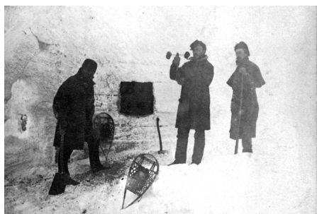
Clough, Smith, and Nelson at the entrance to the weather station —not a door that could be frozen shut by rime and snow, or could be damaged by wind, but a heavy cloth over a small opening in the side of the building.
