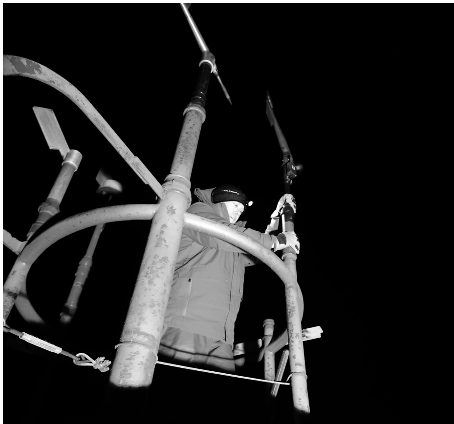
Mount Washington Observatory Staff Meteorologist Ryan Knapp sets an anemometer on the observation tower.
