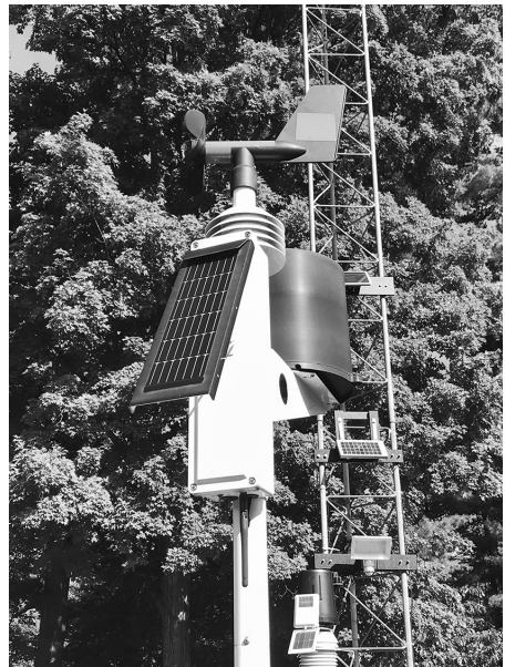
Observations of snow, rain, temperature, sky conditions and more are made by staff and volunteers at the Pine Street weather station.
