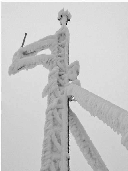
The tower encased in heavy ice conditions.
